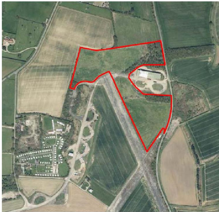
Aerial photograph with application site outlined in red (Courtesy of Bing Maps)
